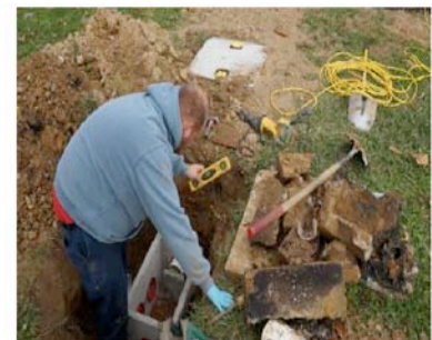
Installation concrete distribution box.
