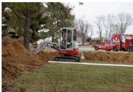
Sewer line installation.
