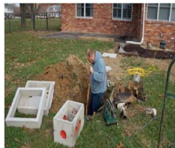
Area prepared for distribution box installation.
