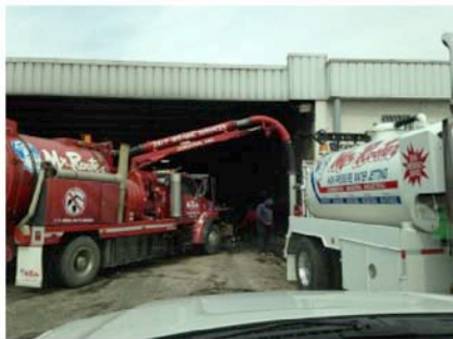
5000 gallon vacuum pumper keeping flow down while line is being cleared.
