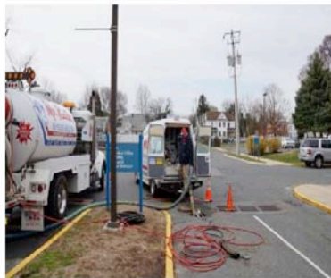
Main line cleaning and video inspection.
