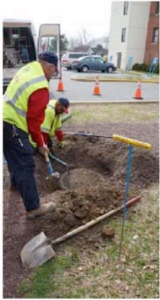
Location and excavation of commercial manhole.
