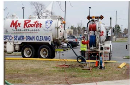
Industrial vac and jetter trucks working to clear main line blockage.
