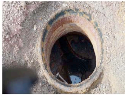
Manhole open and ready for pumping maintenance.
